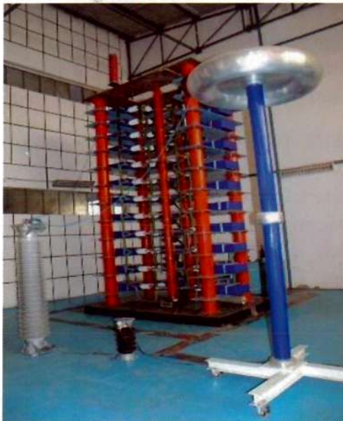
L.I.P.L Test at 20kA on 168kV surge Arrester 176kJ, 840kV IMPULSE GENERATOR
